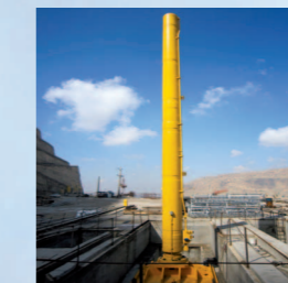
Servomotor for power intake gate
